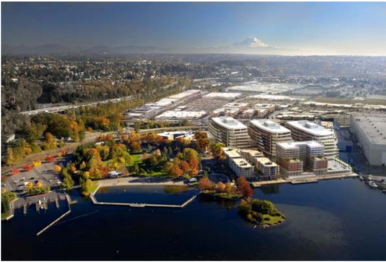
An aerial view of the proposed Southport development.
